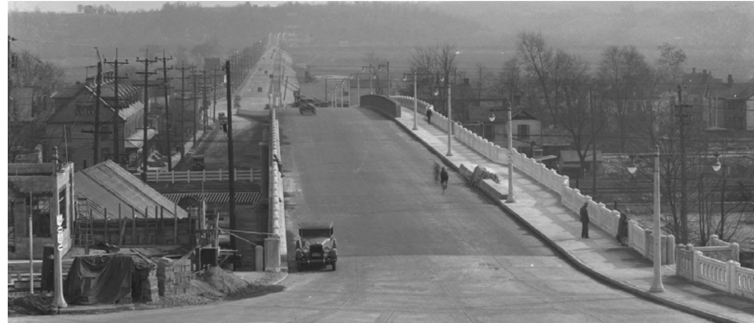
Beechmont Levee 1931, looking east
