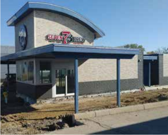
7 Brew Coffee under construction
