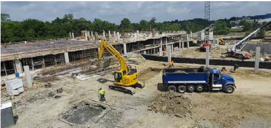
Vantage at Anderson Towne Center Apartments construction in 2023
