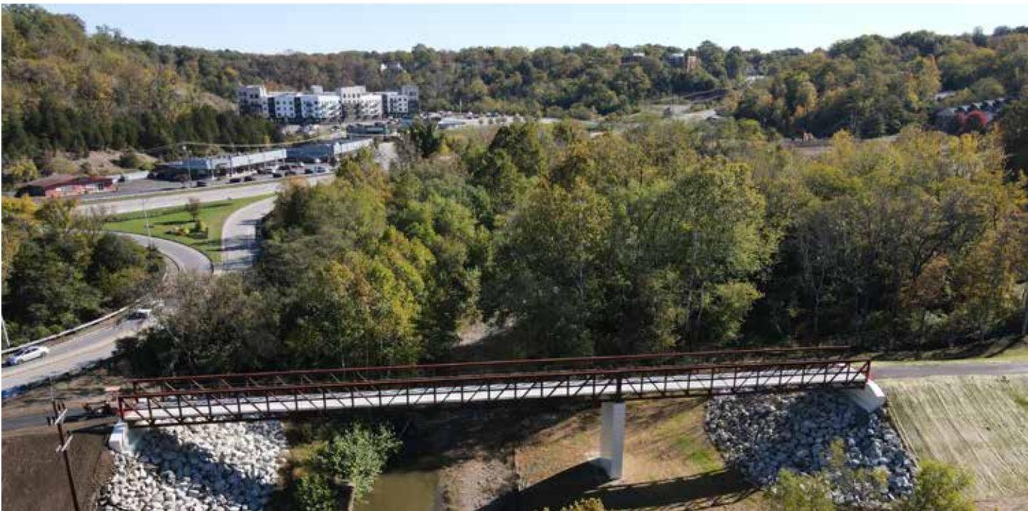
An aerial view of the completed Elstun Connector Bridge over Clough Creek near S.R. 32.
