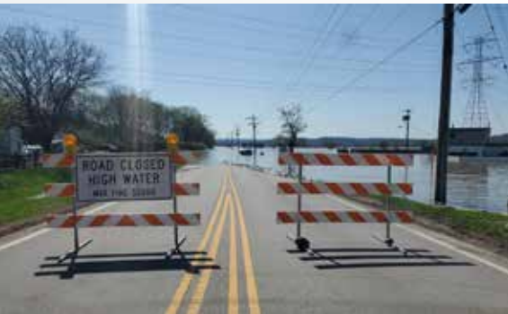
S.R. 32 at Clearcreek Park
